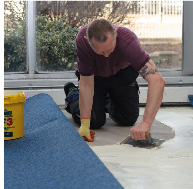
Essentially, the sub floor should be clean, dry and free from contamination such as dust, with any loose material cleaned by scraping, brushing or vacuuming the surface. Contaminants such as paint, residual adhesives, oil, mould or mildew should also be removed using appropriate cleaning products and methods, as they can all prevent adhesives from bonding properly.
